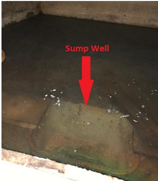
Figure 3: East stair well existing sump well.
